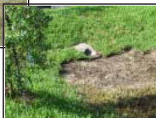
Outfall in swale
