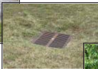
Catch basin in swale
